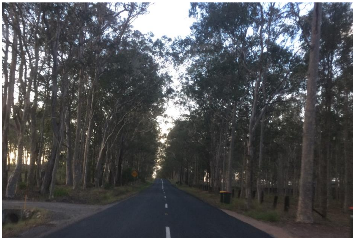
Photo 18– Butterwick Road land widths and shoulders not to Austroad Guidelines
