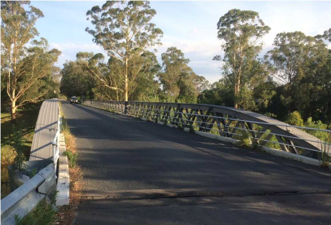
Photo 15–Paterson Road pavement and shoulder widths not to Austroad Guidelines
