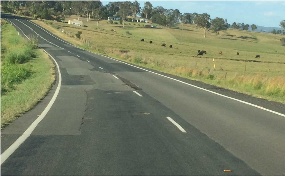
Photo 20– Pavement structural capacity inadequate – Tocal/Maitland Road Paterson
