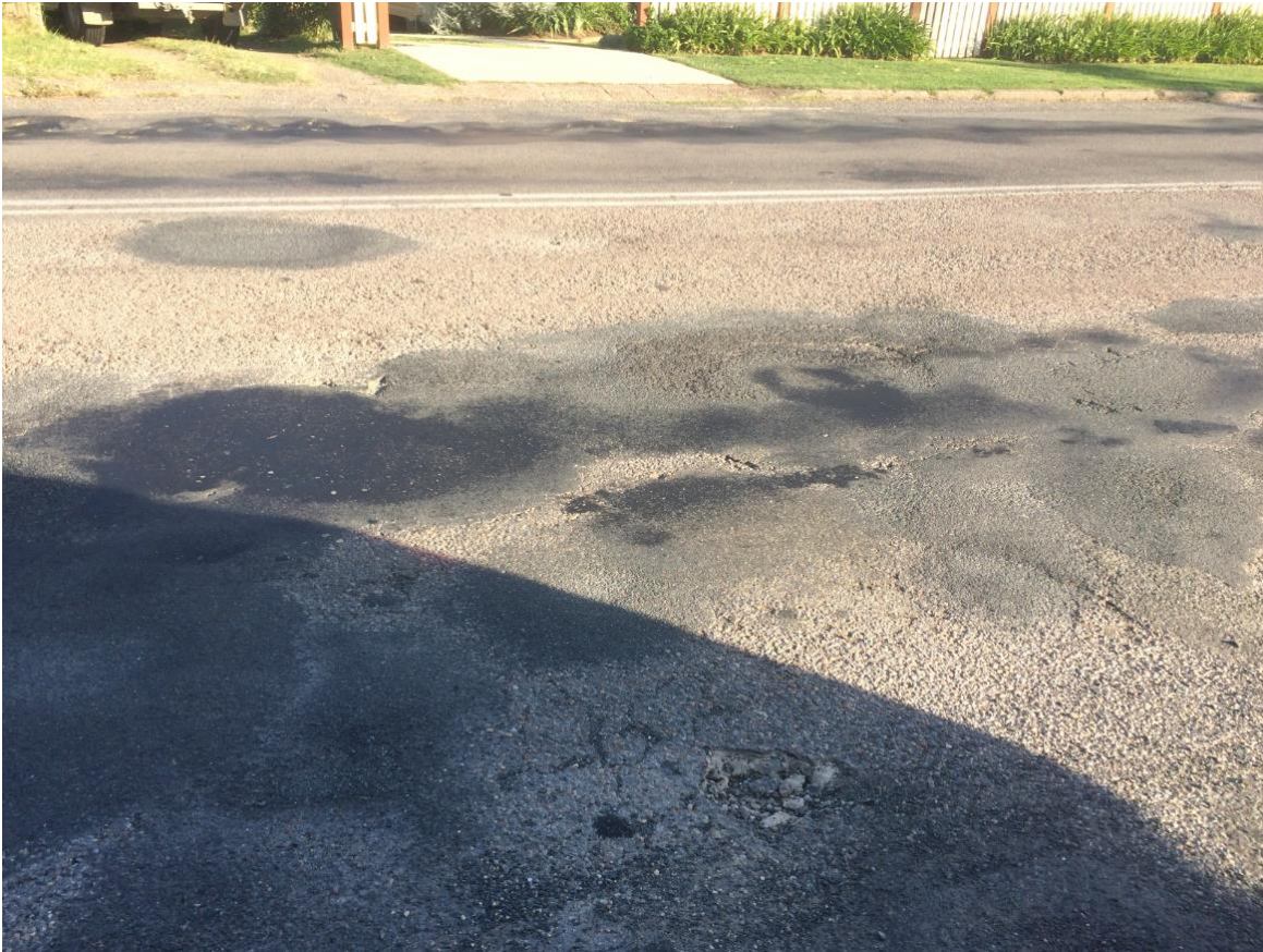
Photo 21– Pavement structural capacity inadequate Tocal/Maitland Road Paterson
