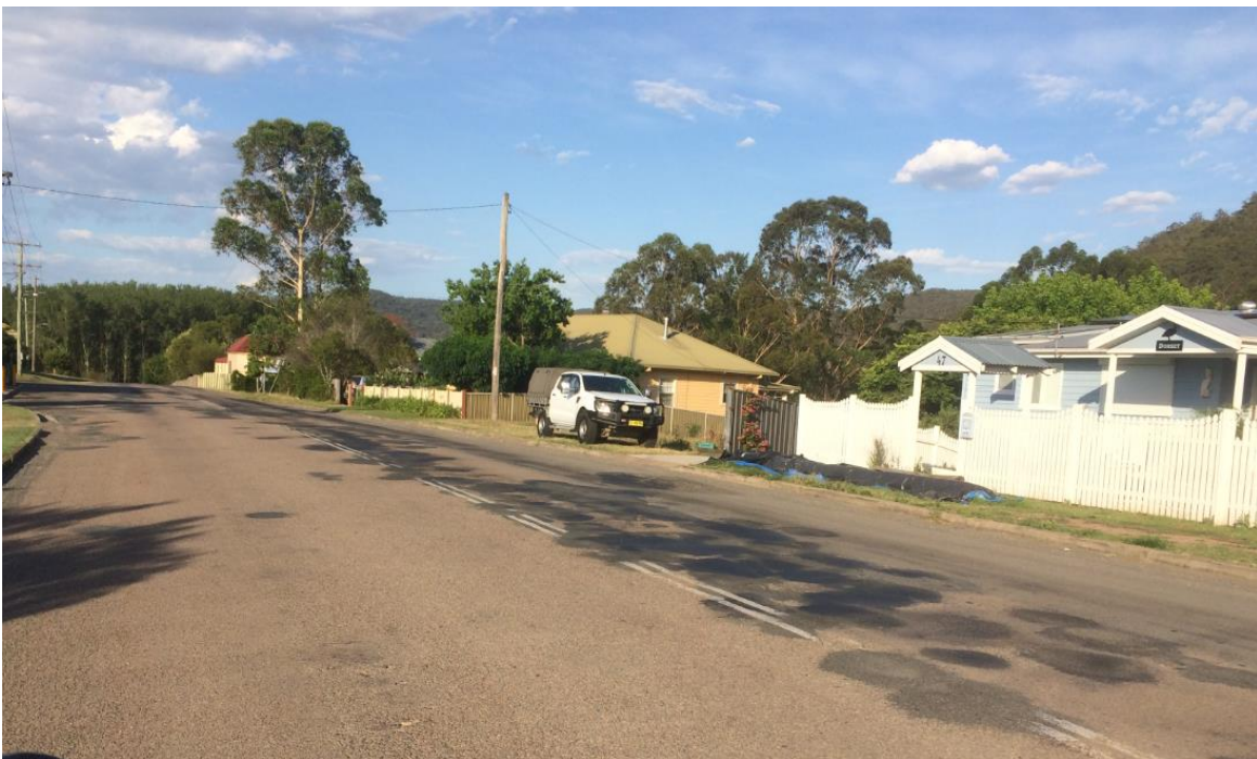
Photo 20– Pavement structural capacity inadequate – Tocal/Maitland Road Paterson
