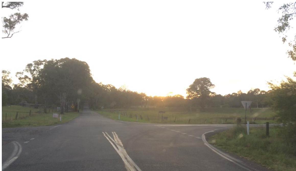
Photo 17–Dunns Creek, Butterwick Road and Paterson Road intersection widths and lanes not to Austroad Guidelines
