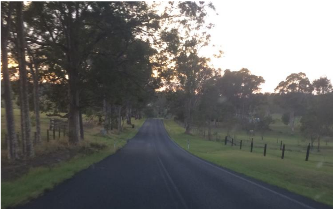
Photo 15–Paterson Road pavement and shoulder widths not to Austroad Guidelines
